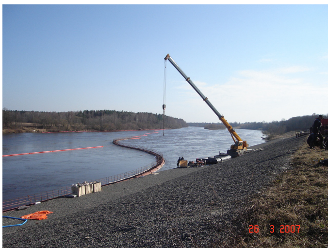
Figure 2.9. The stationary barrier to retain oil on the Zapadnaya Dvina River
